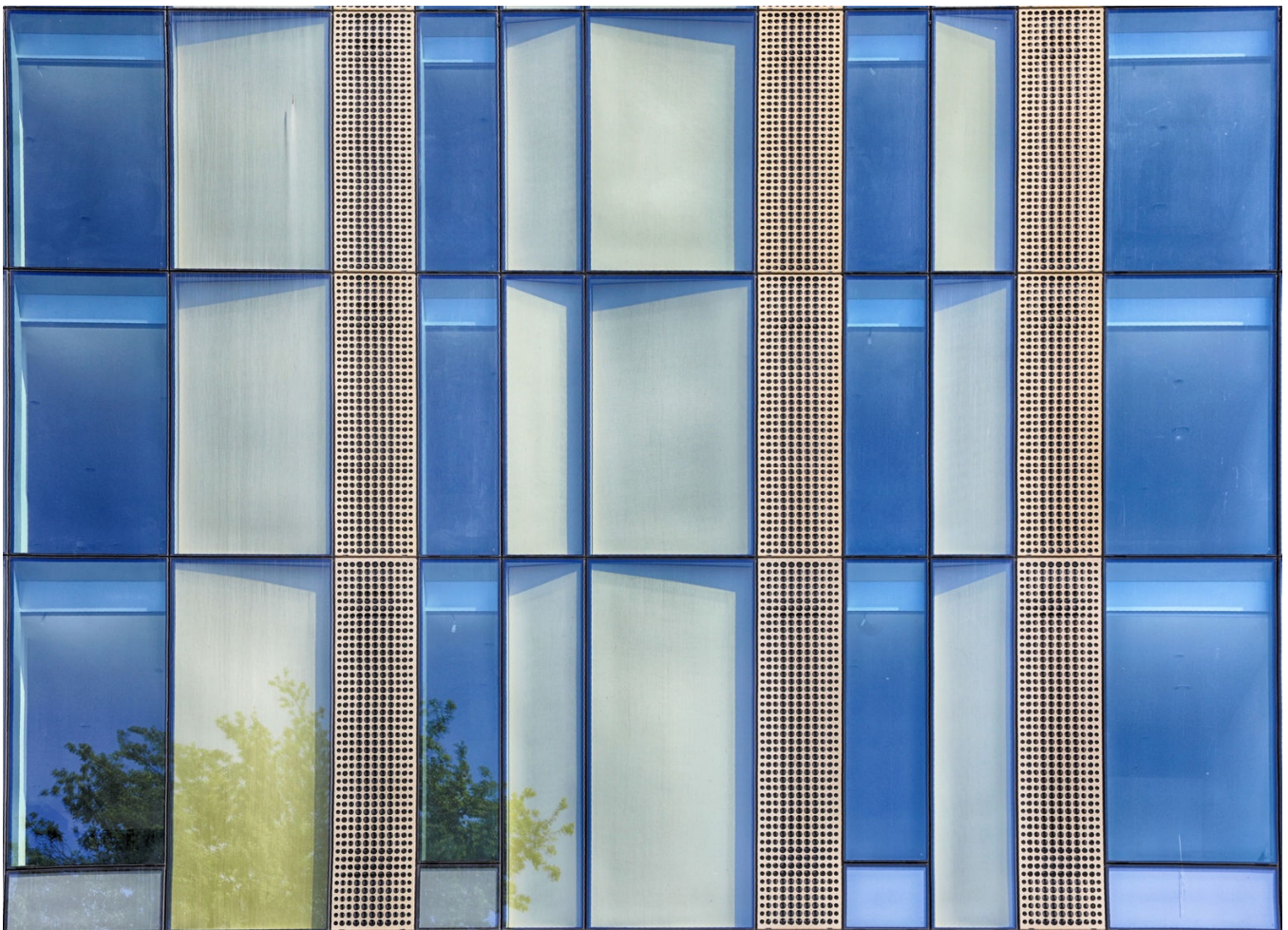
Fig. 3 OMI Architects, Anaconda Cut Building, Manchester (©Courtesy of Focchi).
