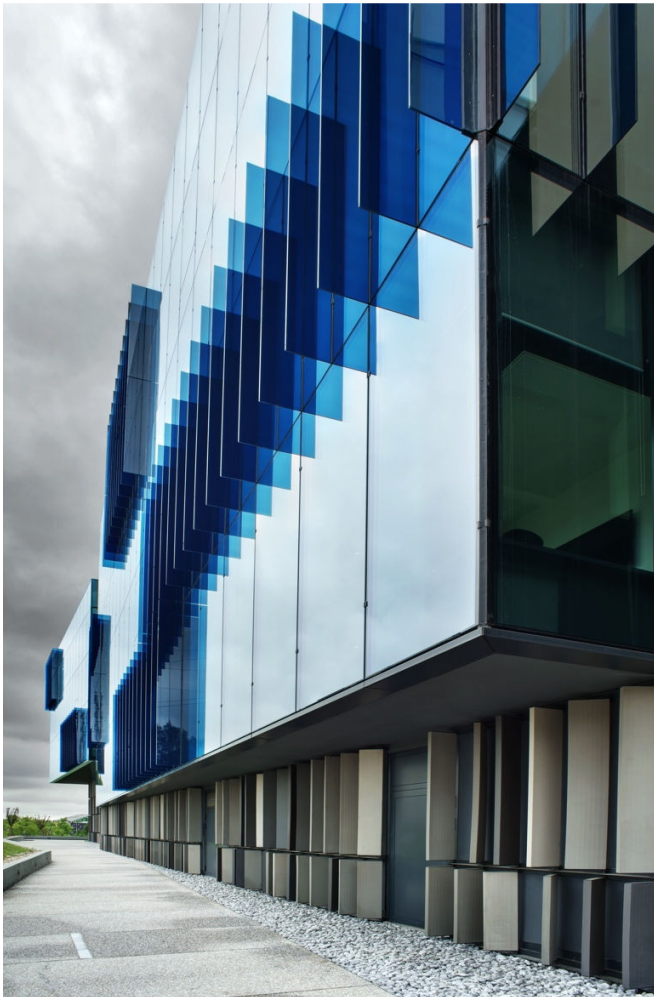
Fig. 8 Park Associati, U 27 Building, Assago (Milan) (©Courtesy of Focchi).
